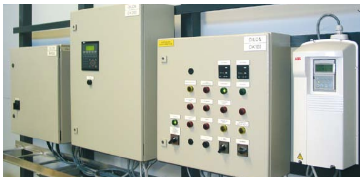
All-inclusive burner automatics: oxygen (O 2 )/pressure differential cascade control
