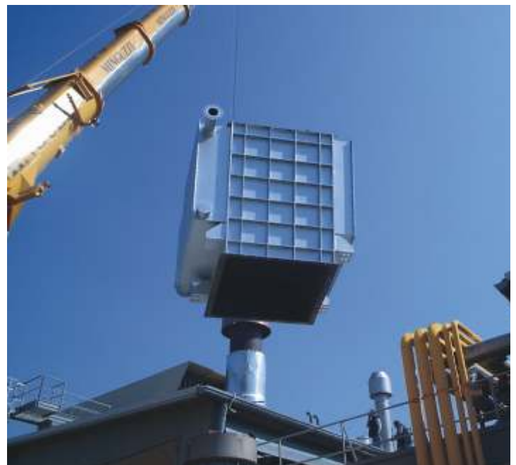
Economizer during site erection
